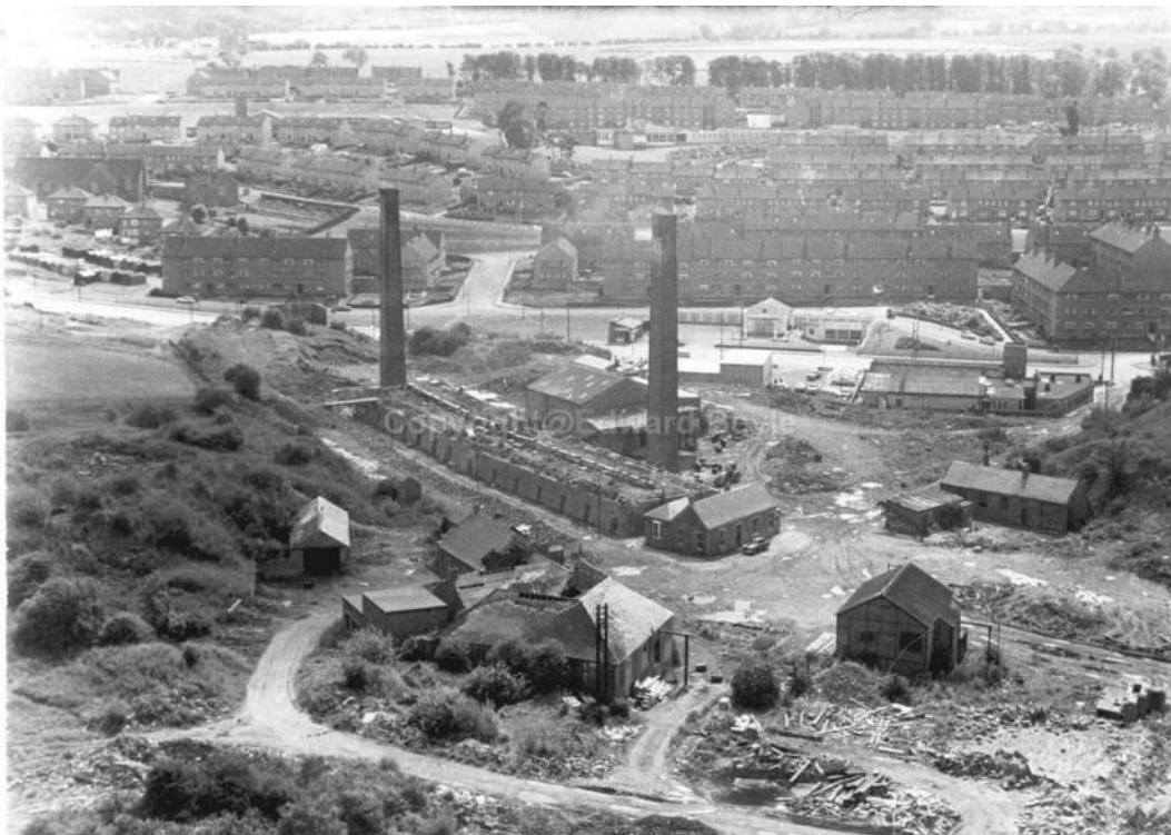
Photograph showing Gateside Brickworks, looking south from the top of the colliery bing. The colliery baths are to the south west at the main road. (Reproduced by permission of Edward Boyle).
